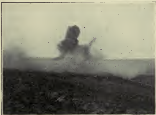
Blowing up of the Oliphant River bridge.
